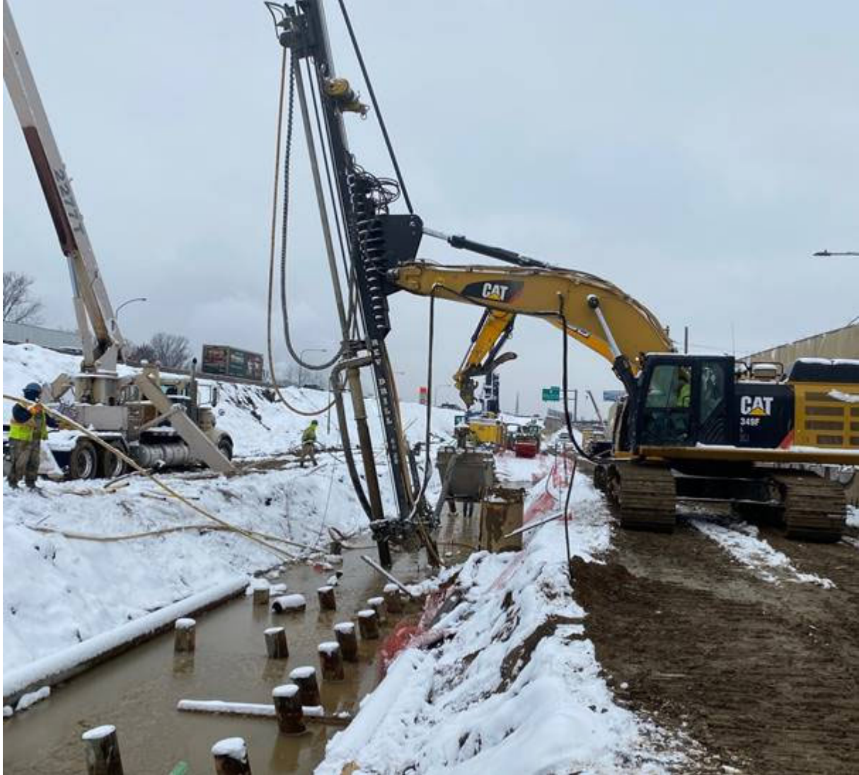
Photo 2) Installing battered micropiles at Wall 3SB.
