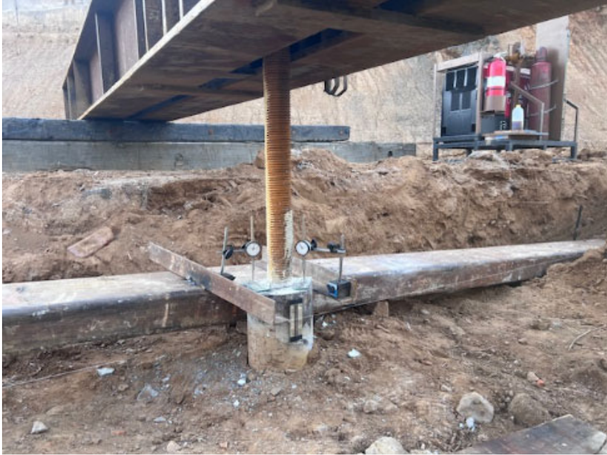
Photo 3) Performing tension load test on sacrificial verification test micropile using No. 28 center bar.
