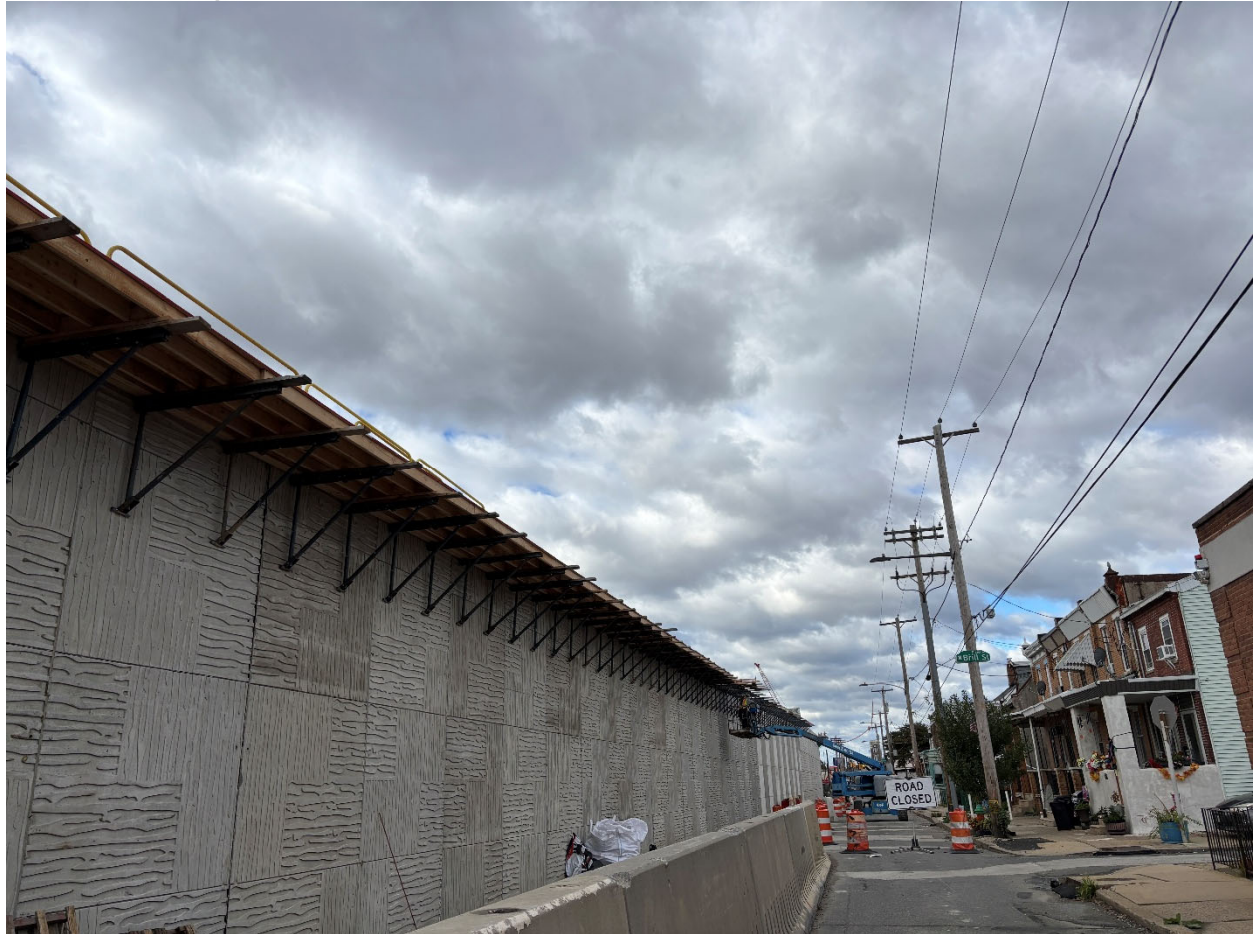
Photo 4) Completed Wall 3SB with architectural finish.
