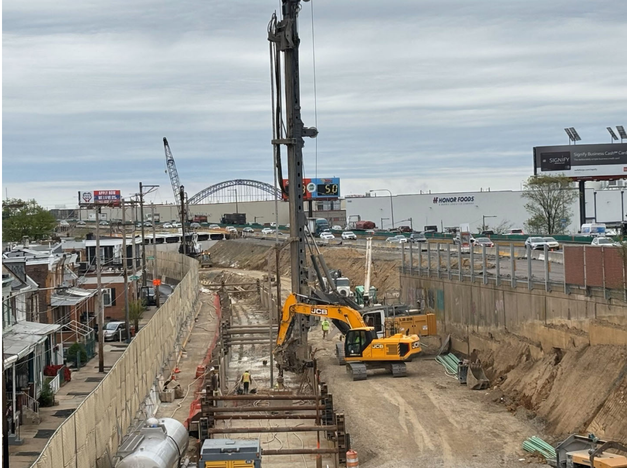
Photo 1) Micropiles installed at Wall 3SB to mitigate impacts on nearby private residences
