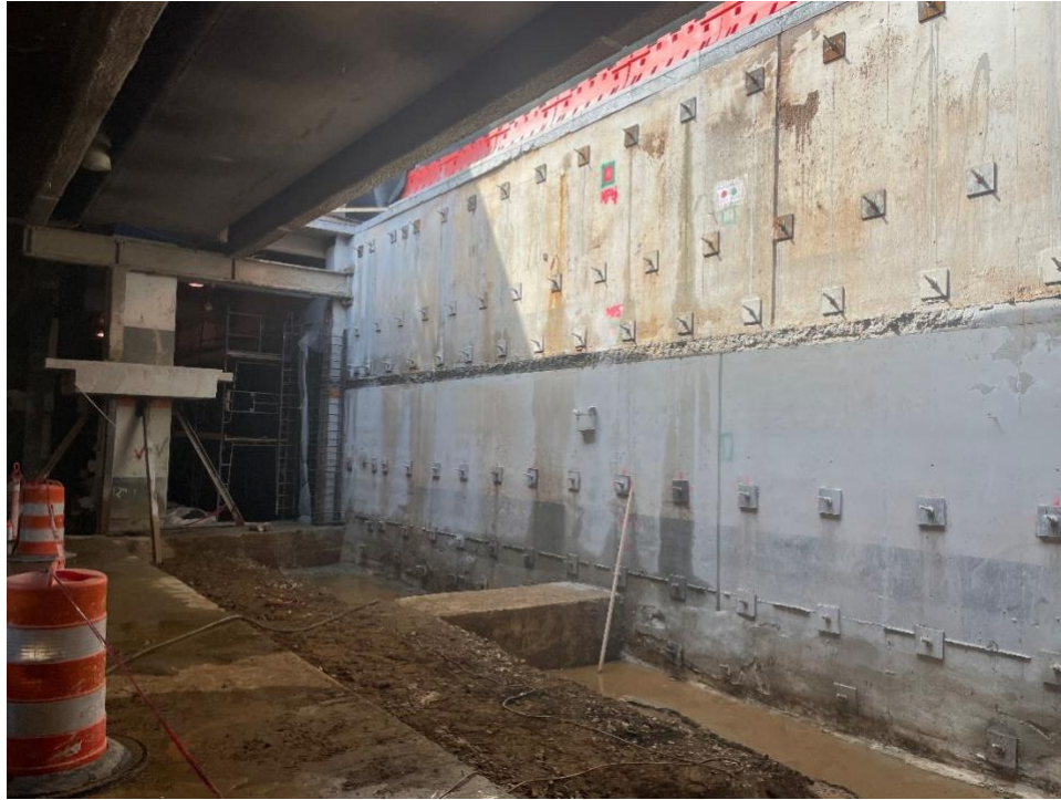
Figure 4: North view of existing foundation wall with floor and roof slabs removed, concrete soldier beams, rock excavation, and temporary SOE construction access ramp. Proximity of adjacent Research Facility and actual work area.
