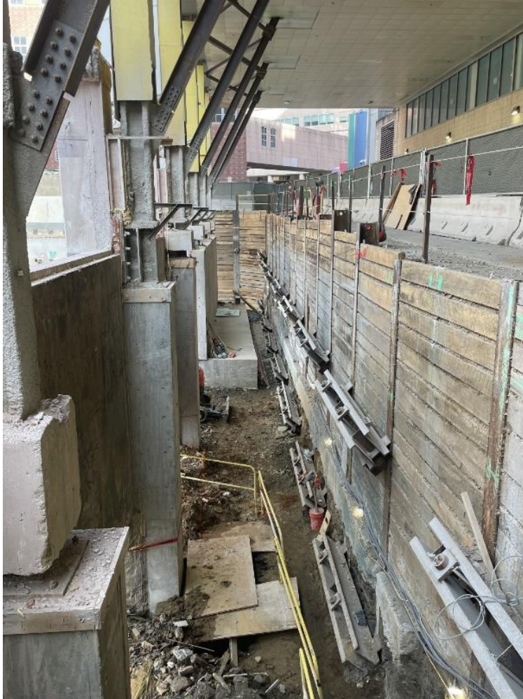
Figure 5: East Service Drive support of excavation in low overhead conditions required steep tieback anchors to clear CHOP Main Hospital basement foundations.
