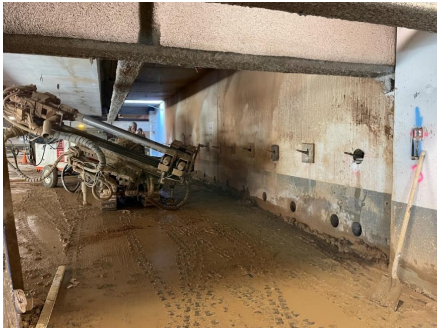
Figure 2: Low overhead clearance inside the existing Osler Garage.
